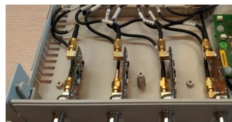
Figure 1. Photograph of external preamplifiers with SAW filters at 298MHz (7T) connected to the adapted digital 1.5T receivers.
